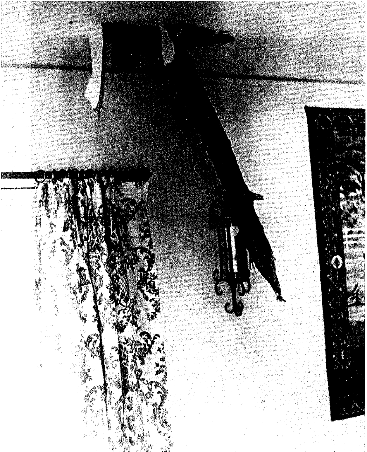
The force of Frederic's 85-knot winds created unusual damages to several of the on-base structures. Among them was this pine timber that was driven through the roof of a base housing unit and into the living quarters.
